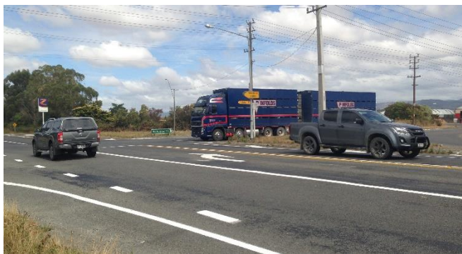
Current Norfolk Road/SH2 intersection
