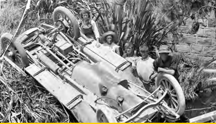
Road safety has been a concern for the AA in Taranaki for all of its 100 years. This photo (PHO2014-0368) from Puke Ariki's photographic collections shows a car accident at the Opuia Bridge near Opunake on February 2, 1914. The vehicle plunged over the side of the bridge, pinning driver Dan Deegan underneath. He was discovered six hours later and rescued, subsequently making a good recovery. Broken steering gear was said to be the cause of the accident.
